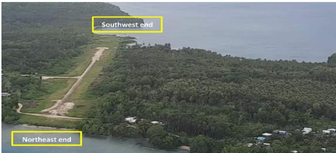
Figure 12: Santa Cruz airport showing both runway ends
