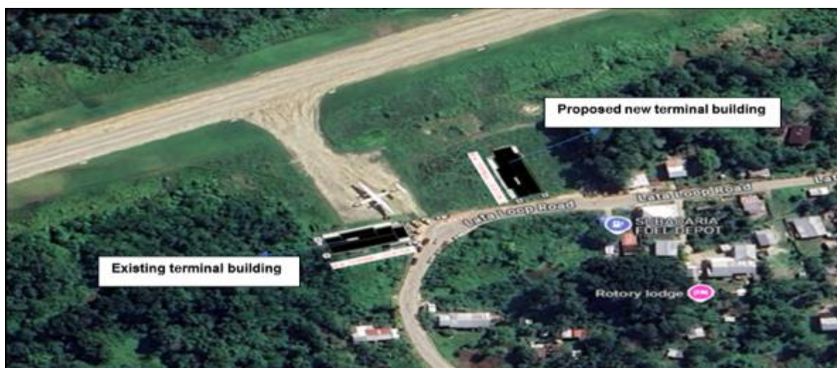
Figure 11: Location of the proposed new terminal building and the existing terminal building
