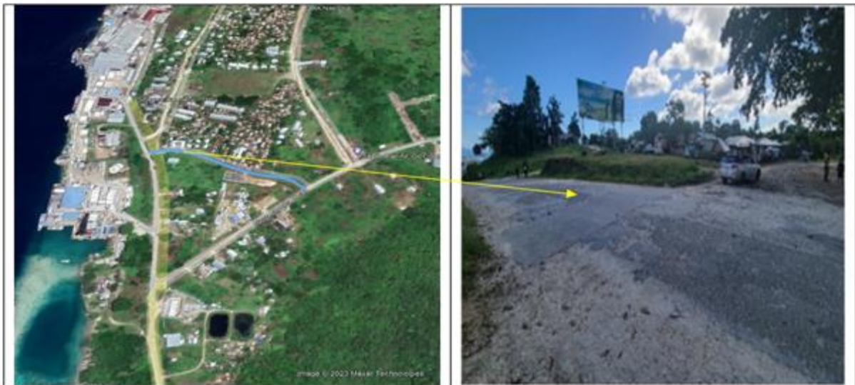
Figure 8: Existing condition of identified Kitano Road
