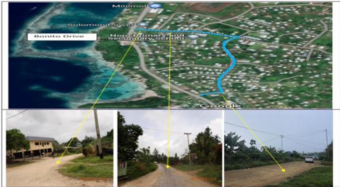
Figure 18: Location and existing condition of Bonito Drive
