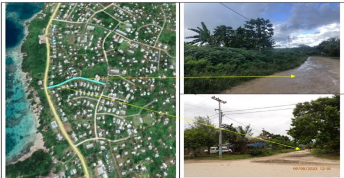
Figure 19: Location and existing condition of Baru Feeder Road
