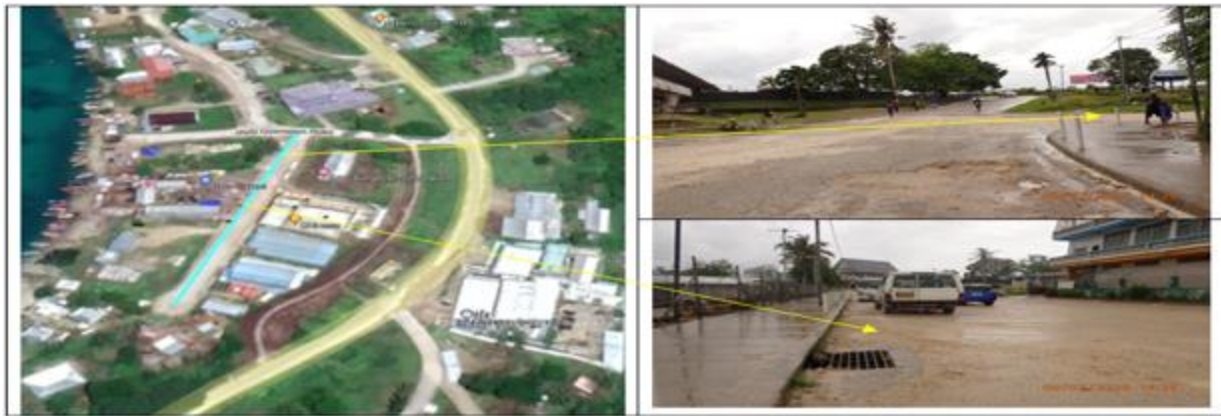
Figure 15: Location and existing condition of Market Road
