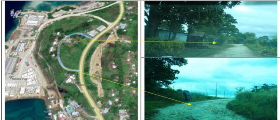
Figure 13: Location and existing condition of Customs Road
