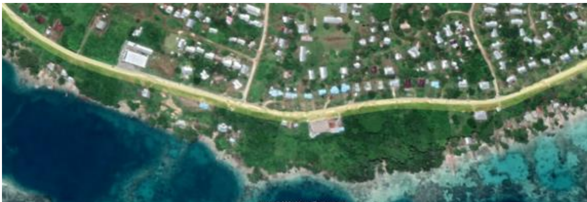
Figure 33: Section of main Noro Highway separated from marine environment by vegetated buffer
