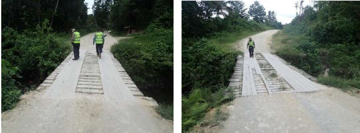
Figure 5: Bio 1 (left) and Bio 2 (right) bridges
