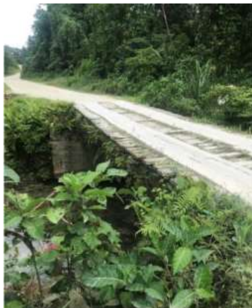
Figure 3: Koa timber bridge without a pedestrian walkway
