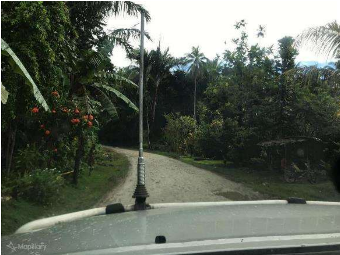
Figure 7: Examples of active use of land within the road reserve up to the shoulder.
