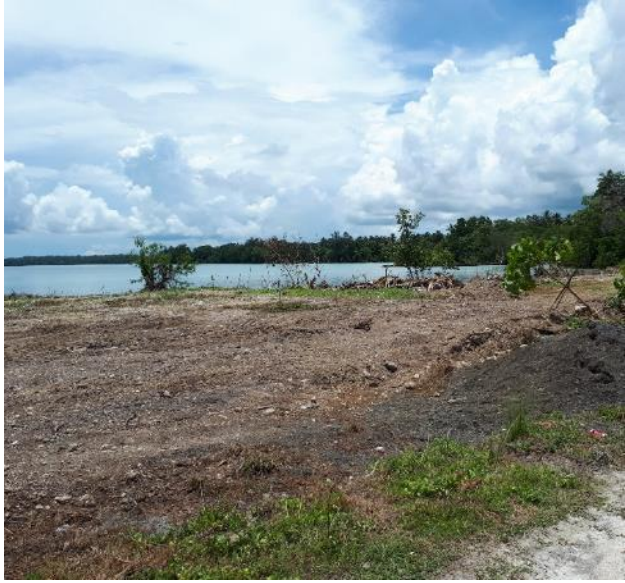
Figure 11: Vegetation clearance western end of MUA runway
