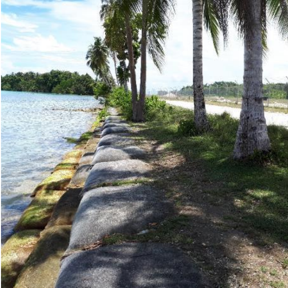
Figure 10: Coastal reinforcements along southern side of runway
