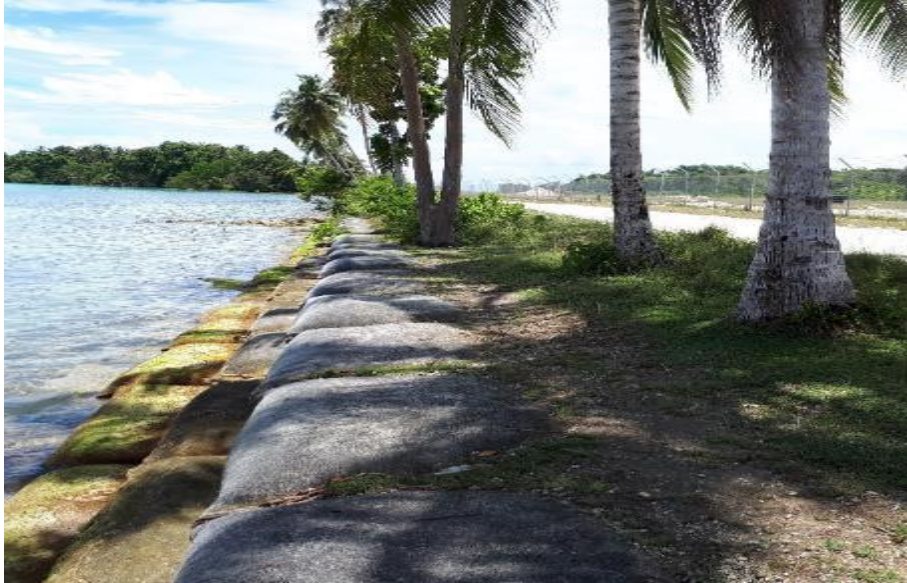
Figure 14: Coastal reinforcements along southern side of runway
