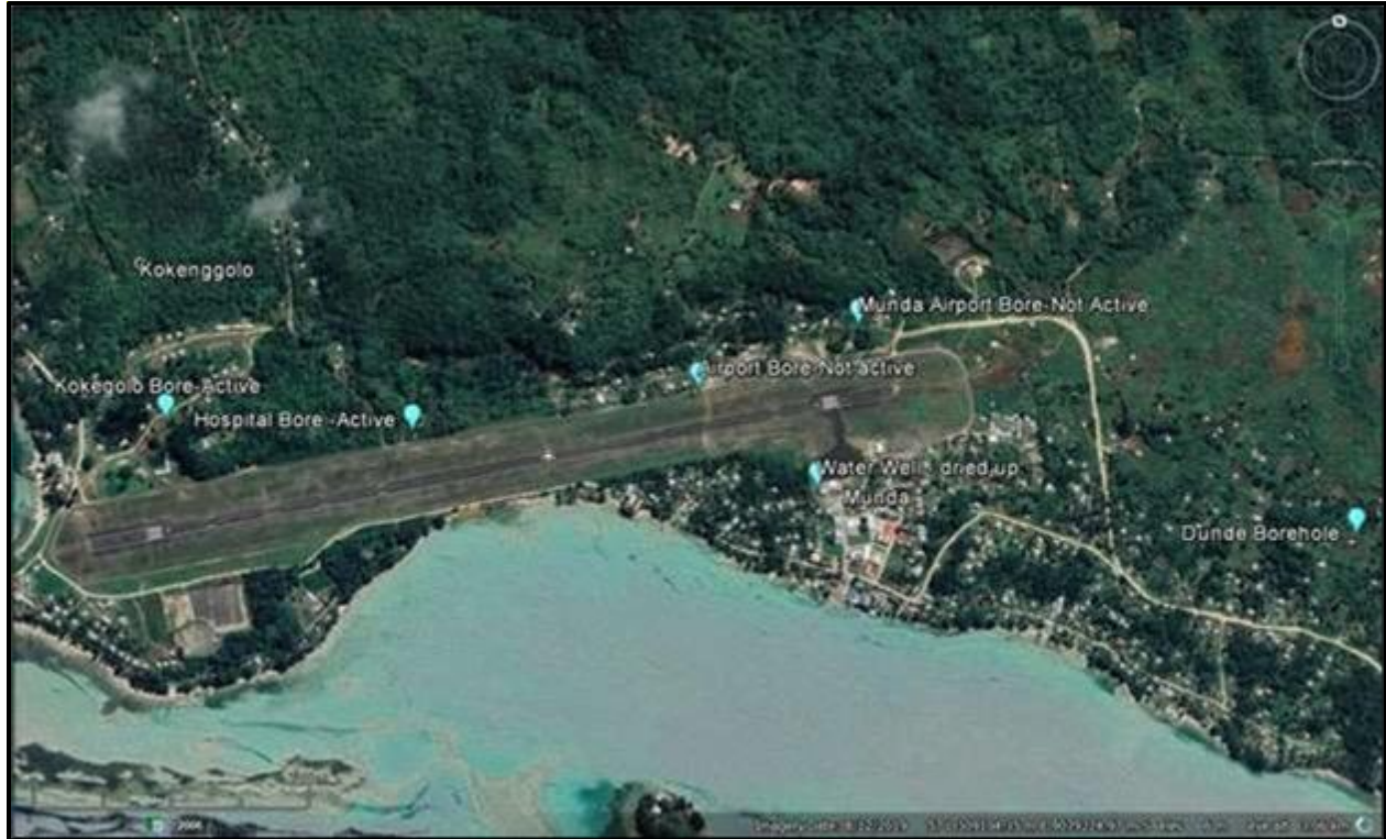
Figure 12: Water supply boreholes in Munda (source from Solomon Water)
