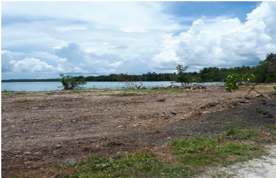
Figure 15: Vegetation clearance western end of MUA runway
