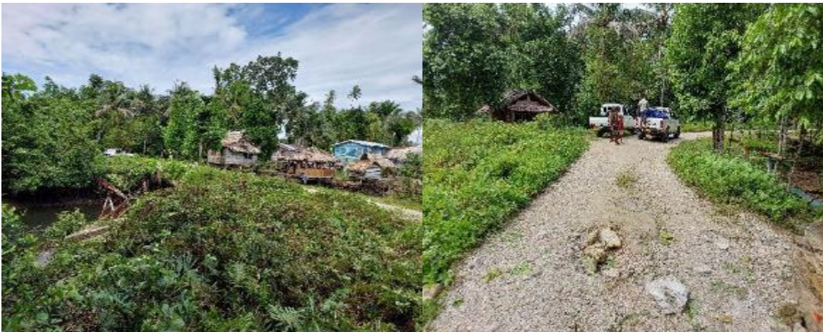
Figure 22: Vegetation cover at bridge site
